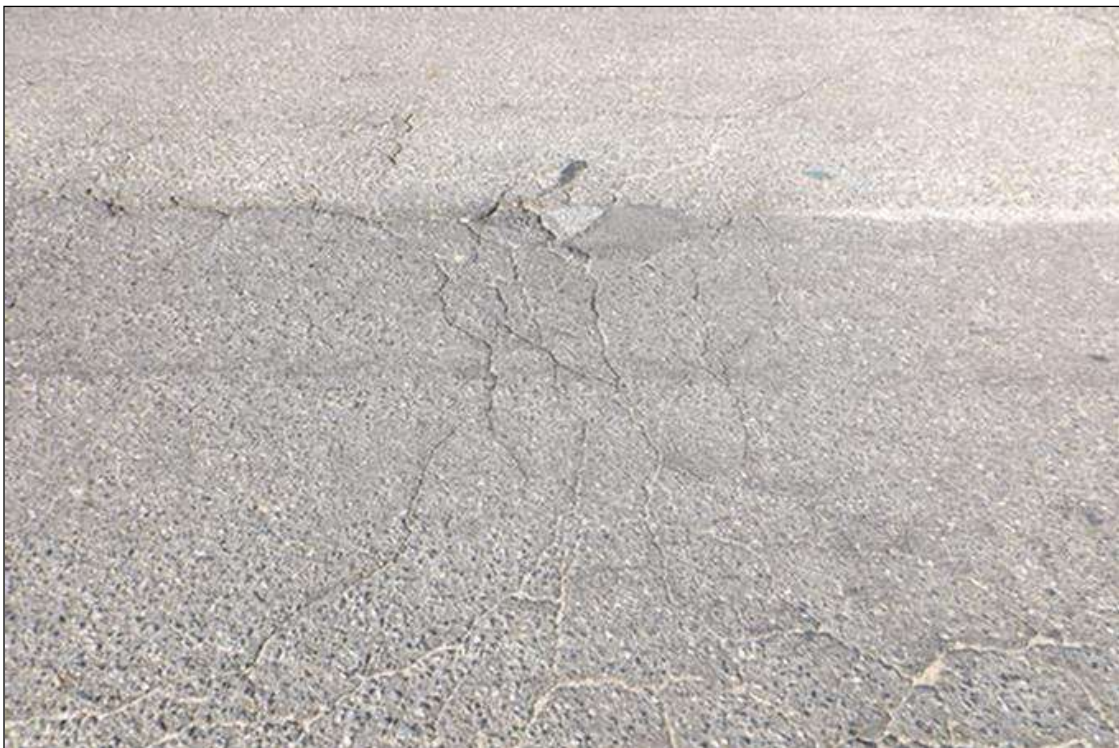
UP TO 1/8" ALLIGATOR CRACKING IN EAST APPROACH ASPHALT WEARING SURFACE
