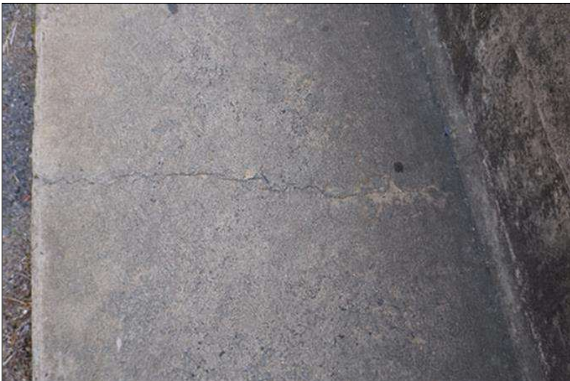
HAIRLINE TRANSVERSE CRACK IN NORTH SIDEWALK (OTHER LOCATIONS SIMILAR)
