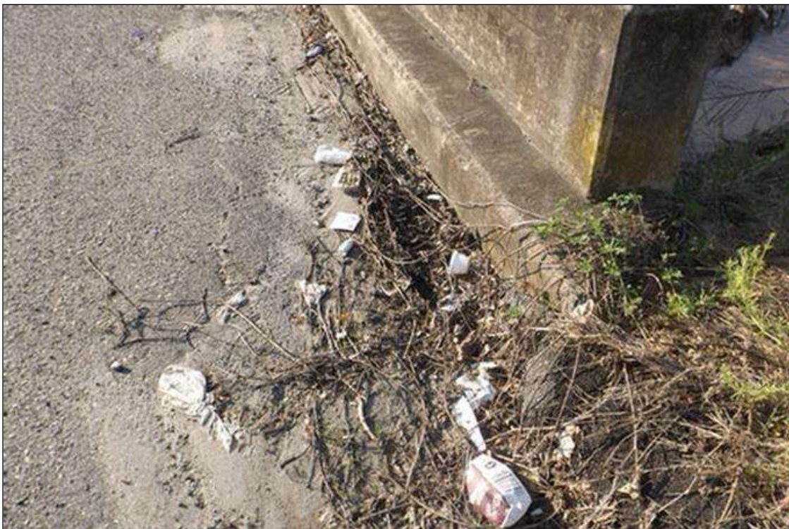
DIRT AND DEBRIS ALONG SOUTH GUTTER
