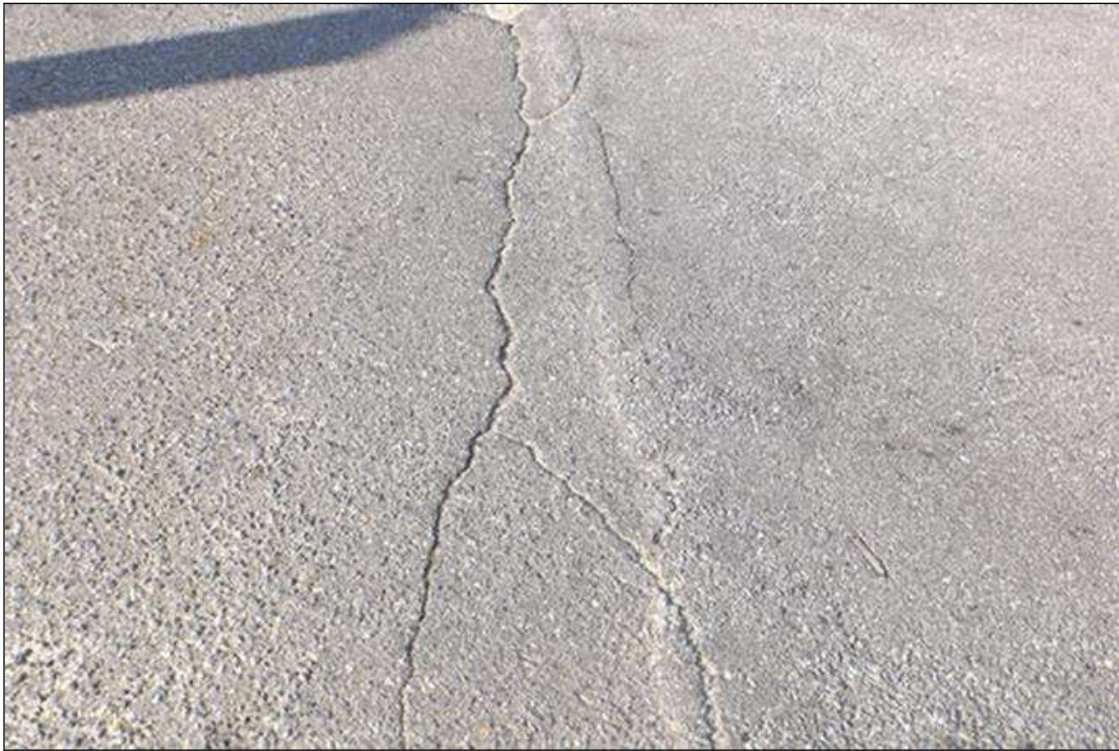
UP TO 1/4" TRANSVERSE CRACK IN ASPHALT WEARING SURFACE AT ABUTMENT 1 (ABUTMENT 2 SIMILAR)
