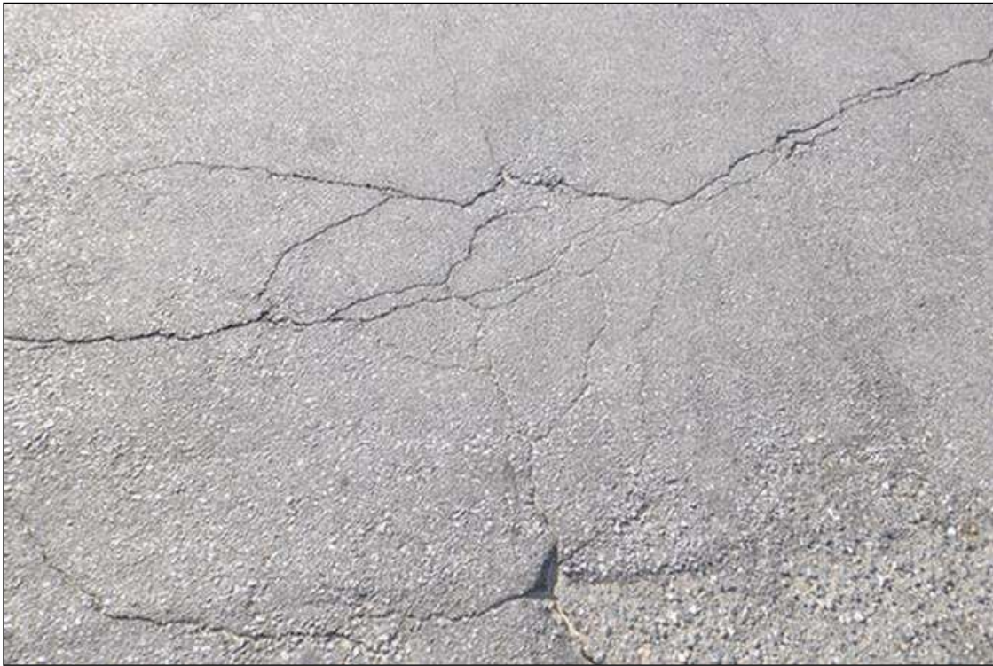
UP TO 1/16" LONGITUDINAL AND TRANSVERSE CRACKS IN WEST APPROACH ASPHALT WEARING SURFACE (EAST APPROACH SIMILAR)
