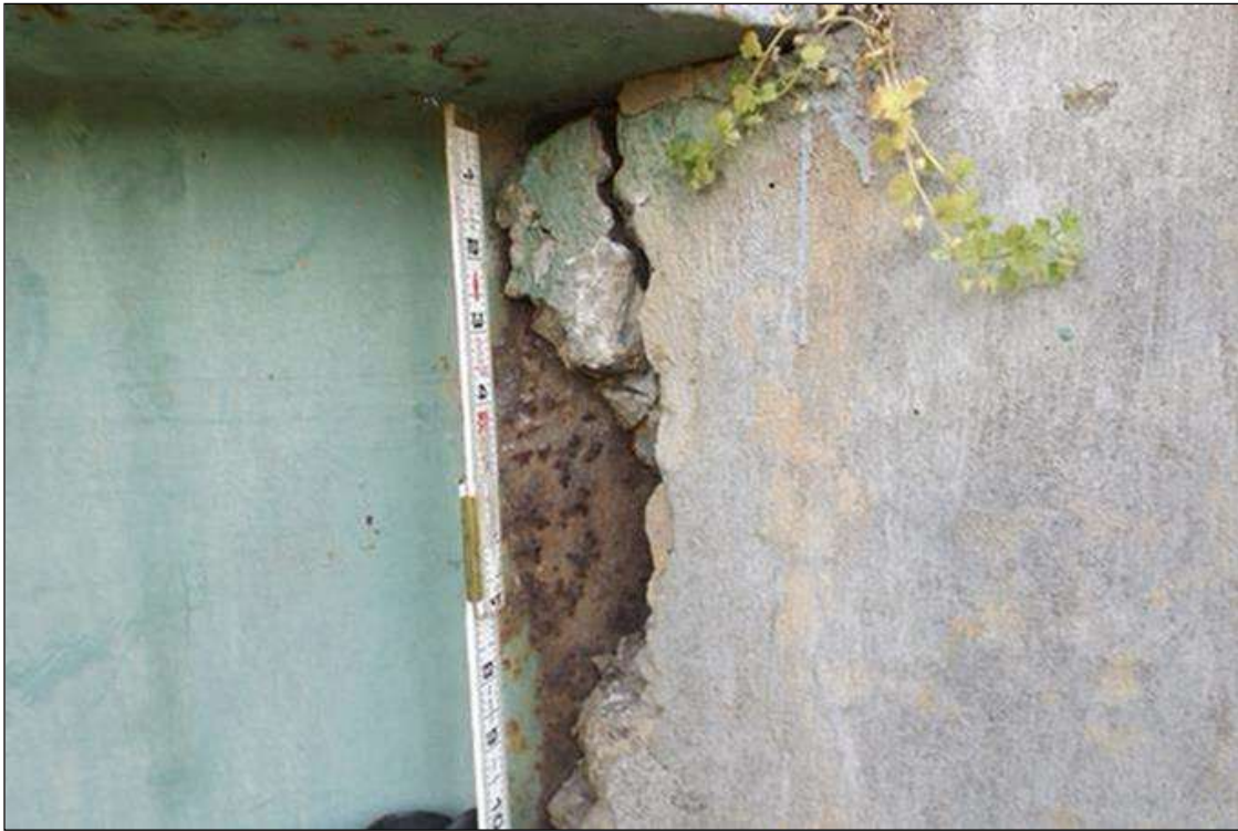
9 1/2" X 3" X UP TO 3" DEEP SPALL IN SOUTH END OF ABUTMENT 2 CURTAIN WALL
