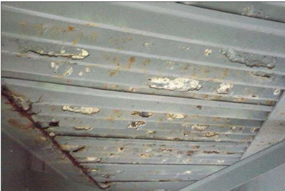
PEELING PAINT AND FLAKING RUST ON STAY IN PLACE FORMS IN BAY 10 (OTHER LOCATIONS SIMILAR)
