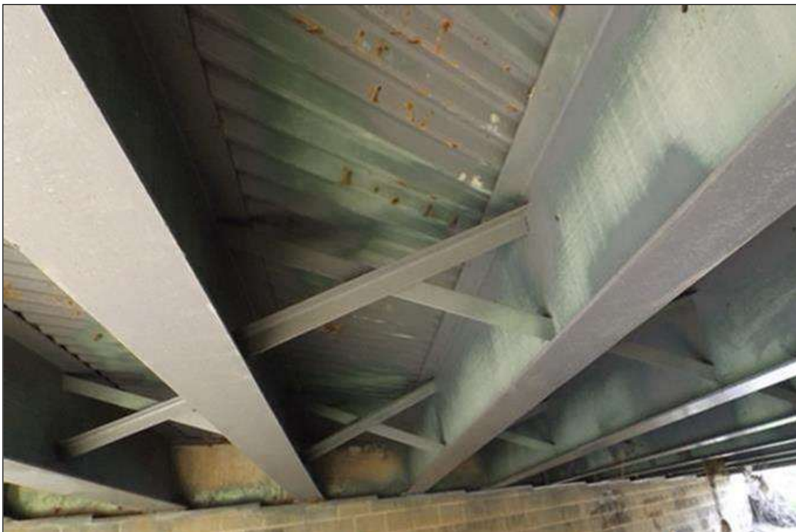
INTERMEDIATE DIAPHRAGM
