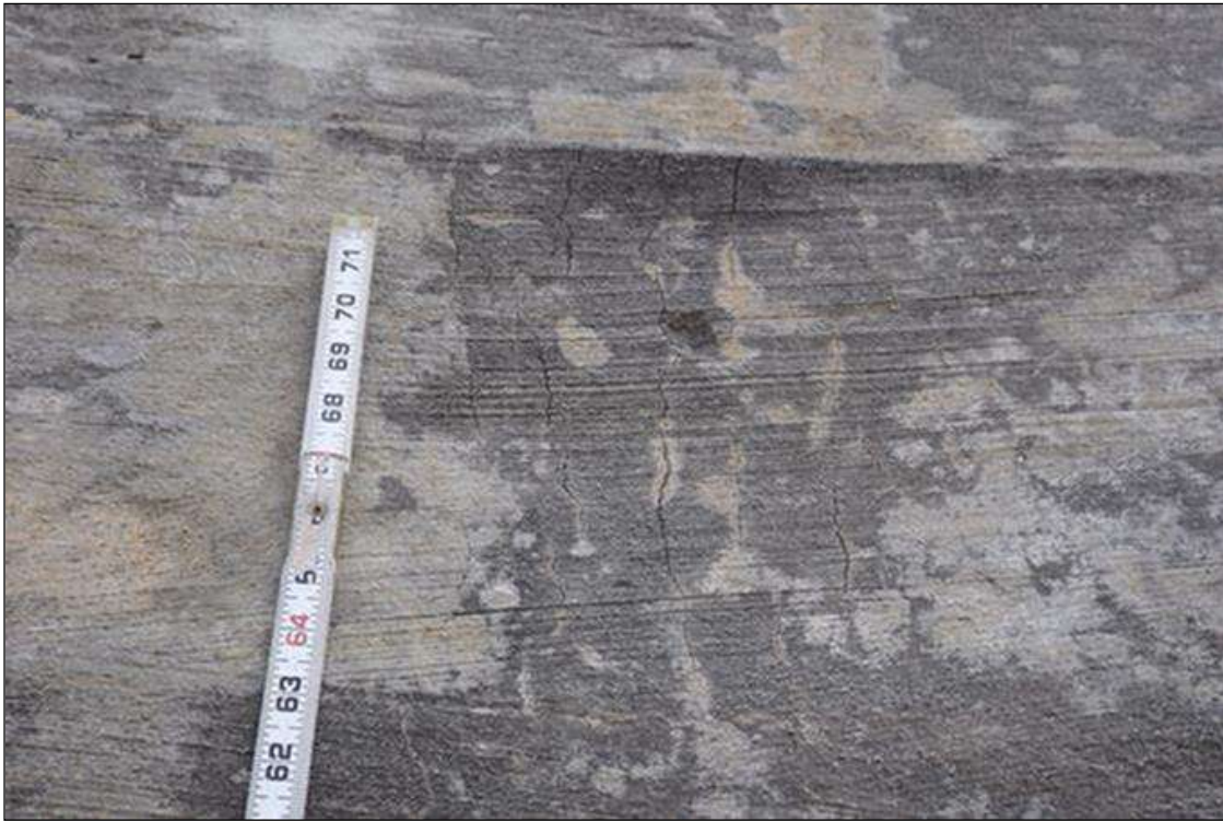
HAIRLINE VERTICAL CRACKS ON OUTSIDE FACE OF SOUTH BRIDGE RAIL
