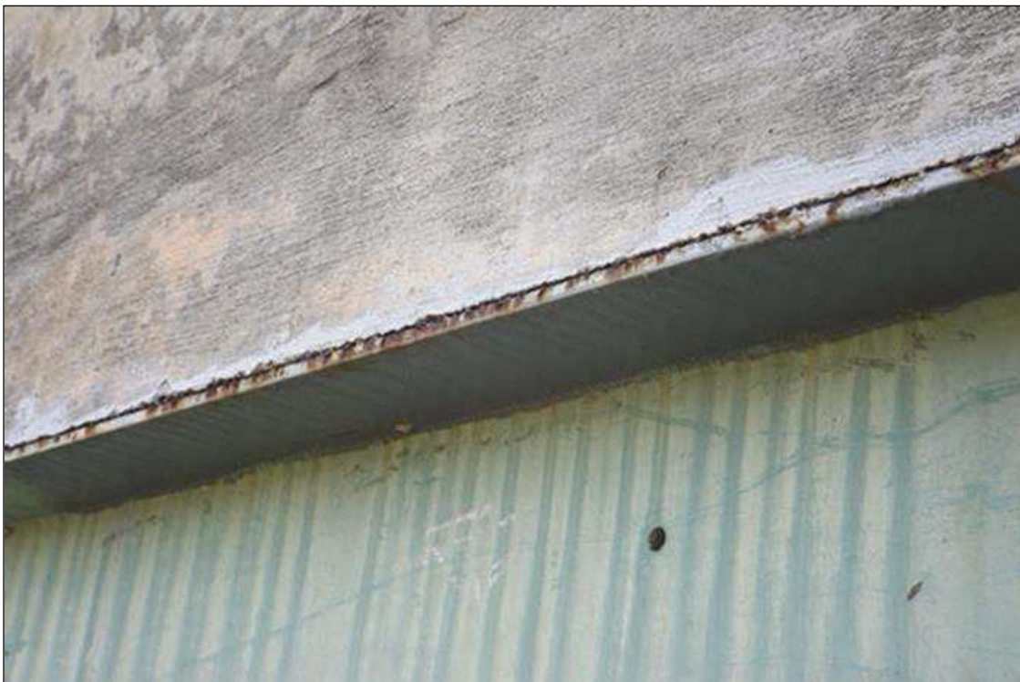
SURFACE RUST ON TOP FLANGE OF BEAM 11
