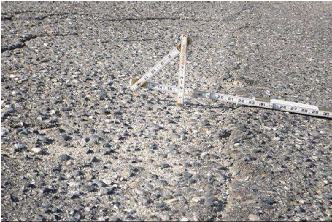
1.5" SETTLEMENT AT EAST APPROACH (SIMILAR AT WEST APPROACH SIMILAR)
