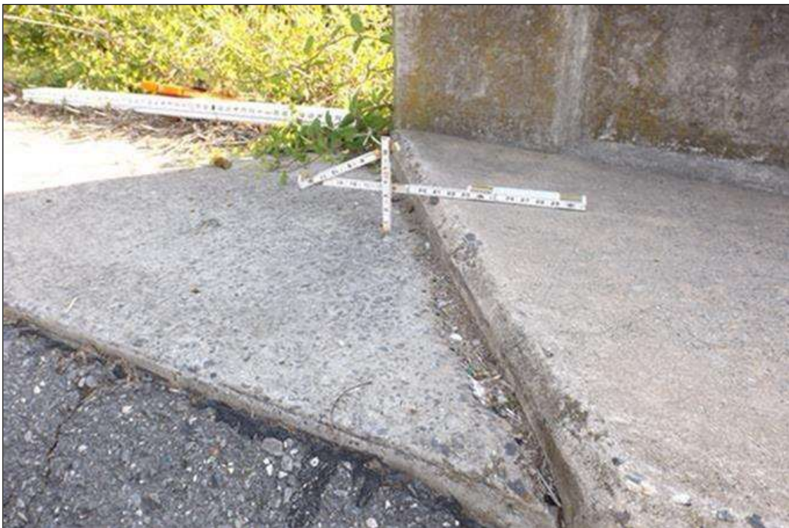
3" SETTLEMENT IN SIDEWALK AT NORTHWEST CORNER (NORTHEAST CORNER SIMILAR)
