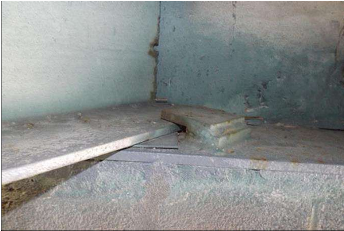
ABUTMENT BEARING (BEAM 6, ABUTMENT 1 SHOWN)
