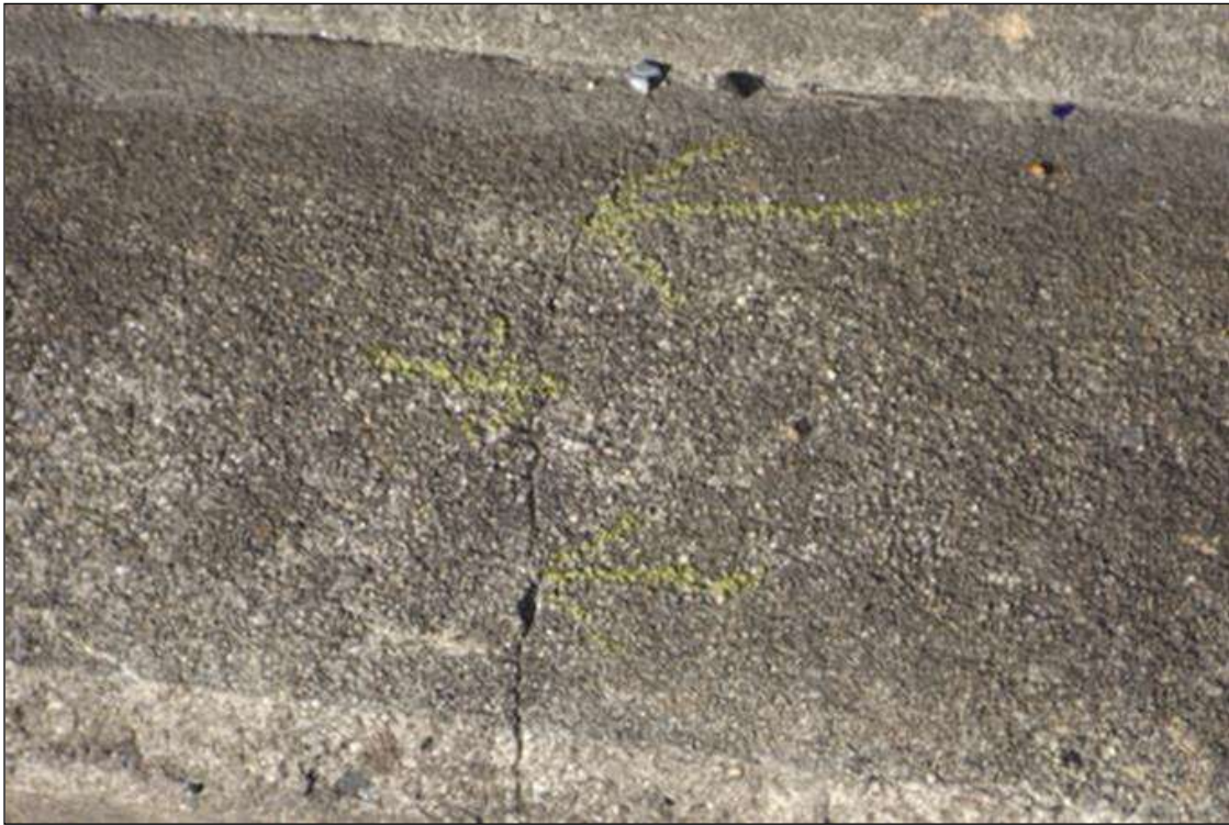
HAIRLINE TRANSVERSE CRACK IN SOUTH CURB (OTHER LOCATIONS SIMILAR)
