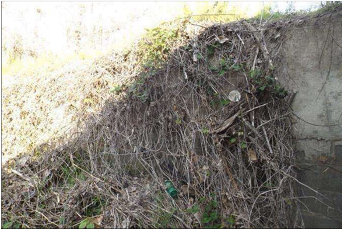
VEGETATION GROWTH ON SOUTHWEST WINGWALL (NORTHWEST AND SOUTHEAST WINGWALLS SIMILAR)
