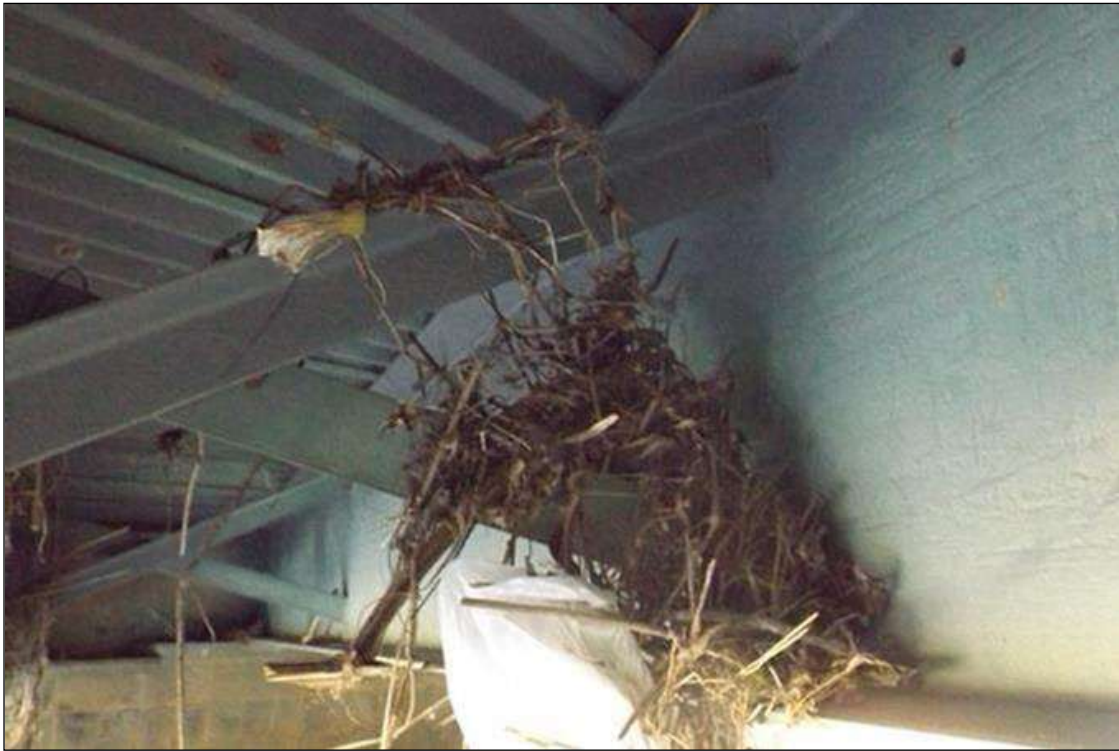
DRIFT ON BAY 8 INTERMEDIATE DIAPHRAGM (BAYS 5, 7 AND 8 SIMILAR)
