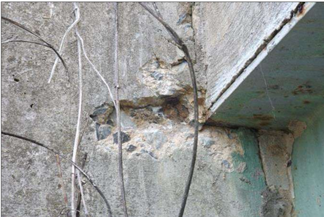
7" X 3" X 1" DEEP SPALL ON SOUTHWEST WINGWALL
